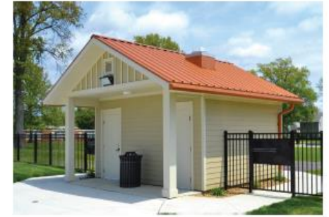
RESTROOM EXAMPLE: ELYRIA, OH
