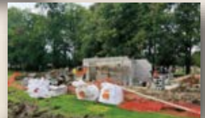
Restroom & Pavilion at John Glenn Park
